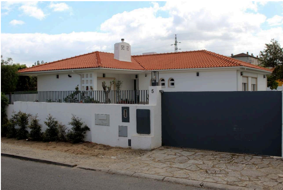
Figure 12. Single-Family DETACHED HOUSE for the senior staff neighborhood, type C. Current view from the street, with one of the multi-family blocks in the background
