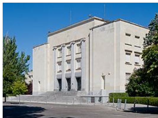
Architecture school. Polytechnic University of Madrid. Avenida Juan Herrera, 4; Madrid
